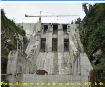
Parbati-II concrete dam under construction, H.P., India
